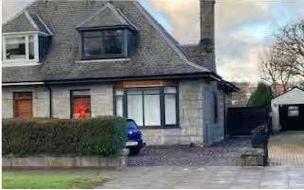
Photo 4: Demonstrating that 56 Cromwell Road has removed a wide section of the low-lying granite wall in order to create a car park to the front of the property.
