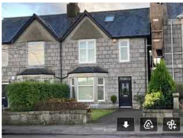
Photo 10: Demonstrating that 25 Cromwell Road (to the immediate left of the Appellant's property) has removed a portion of low-lying granite wall to construct a car park.
