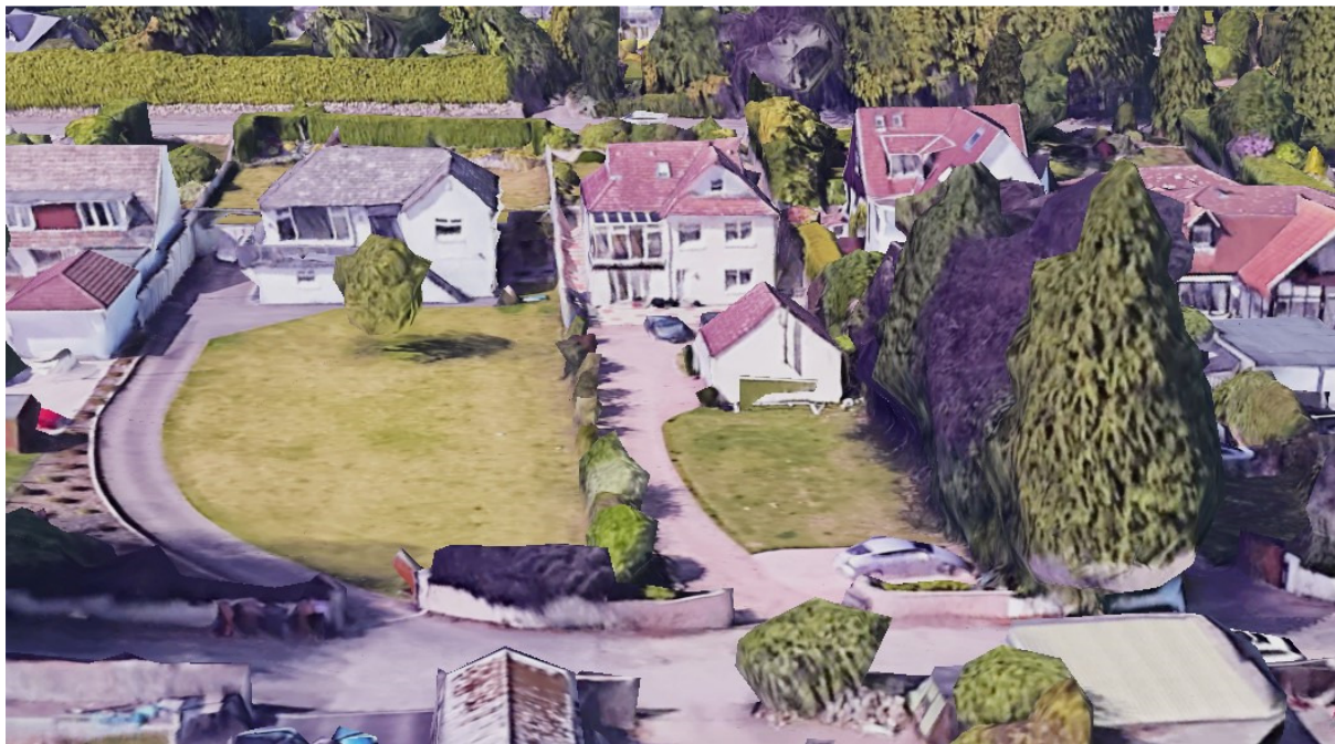
View of No. 25, No. 27 & No. 29 looking North from access lane
