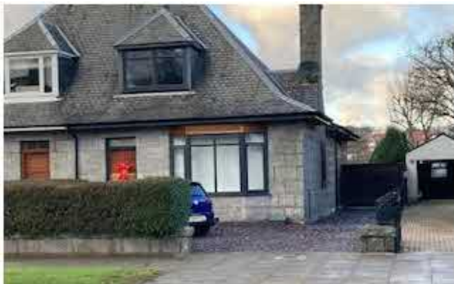
Photo 4: Demonstrating that 56 Cromwell Road has removed a wide section of the low-lying granite wall in order to create a car park to the front of the property.
