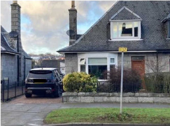
Photo 5: Demonstrating that 58 Cromwell Road has removed a section of low-lying granite wall in order to create a car park to the front of the property.
