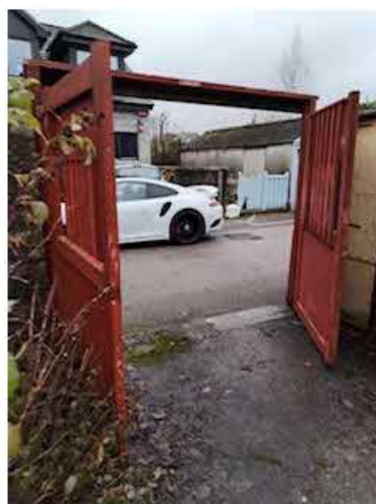
Photo 30: Demonstrating how easy it is to block access to the rear gate of Appellant's property whilst remaining legally parked in the narrow back lane.
